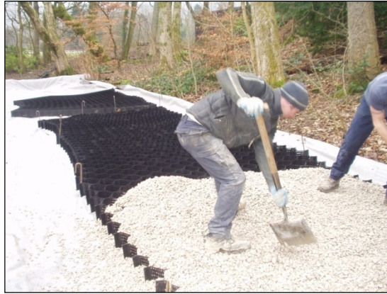
Photo 3- expanding and filling the Cellweb system
