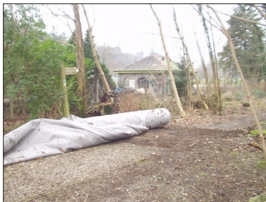
Photo 2- laying of Fibretex material onto existing subgrade
